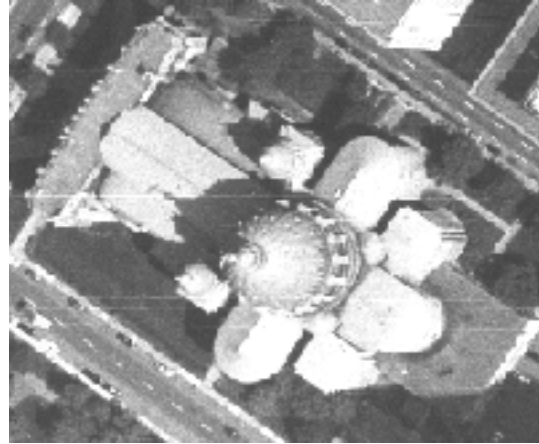
Figure 2.3: Photographic detail of the building in Figure 2.2
