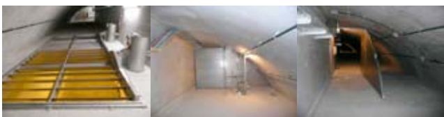
Figure 11: Fresh-air injection device: damper (left), blocking element closed (centre), blocking element open (right) [2]
