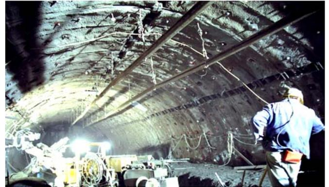
Fig 12. Three rows of yielding elements installed in the shotcrete lining at the Semmering base tunnel
