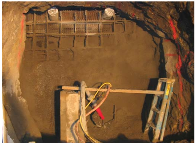
Fig. 5. Bulkhead conditions during construction (note vent pipes at top of bulkhead).
