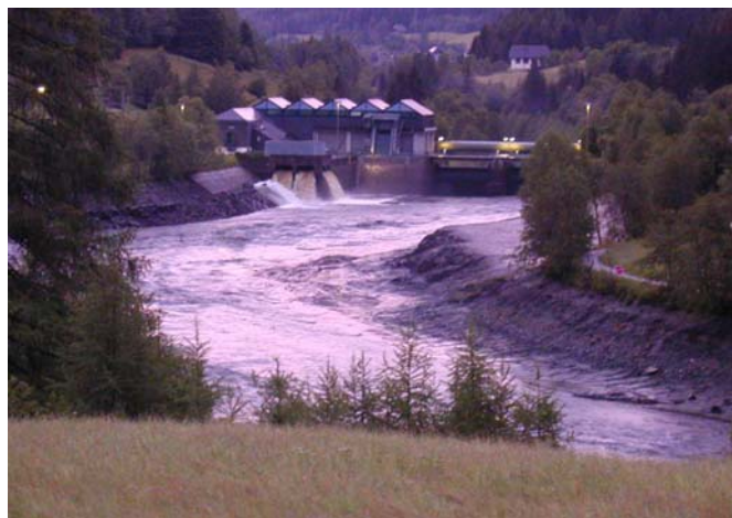
Figure 2 Bodendorf Power plant during flushing
