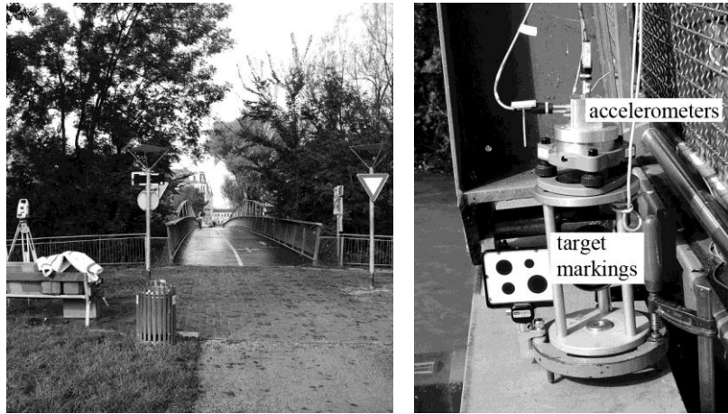
Figure 8. Augarten footbridge equipped with passive target markings and accelerometers for reference measurements.
