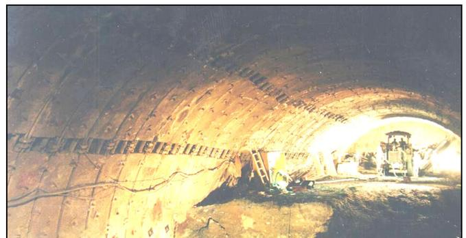
Fig. 1. Galgenbergtunnel Austria; modified support system with integrated yielding steel elements.
