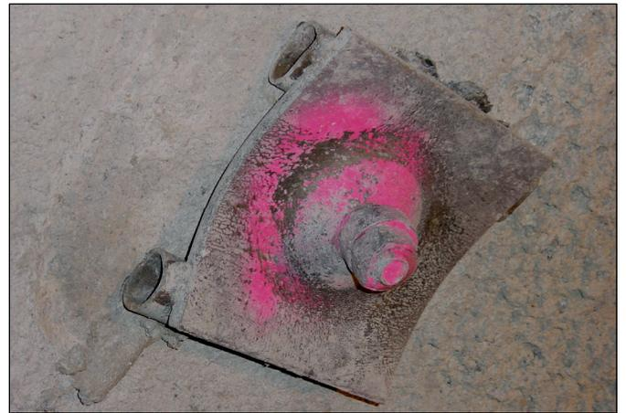
Fig. 6. Deformations on the bolt plate and pipe bridge bearing.
