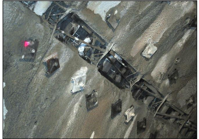
Fig. 5. Lining Stress Controllers in combination with deformable bolt plates at the Strenger Tunnel in Austria [6].
