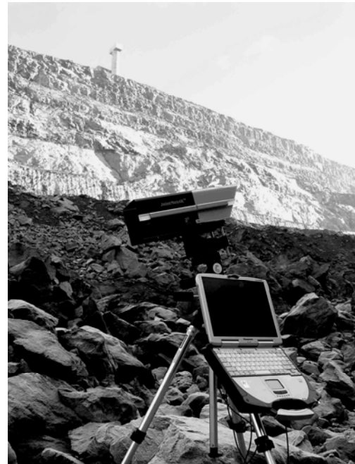
Figure 8: The footwall of the Aitik copper mine from a depth of around 350 m. The ultimate depth will be at 500 m. In the background several block failures affecting bench stability can be observed. The entire slope has to be designed for large scale failure.
